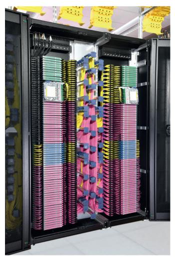
At the heart of the HUBER+SUHNER LiSA high-density fibre management system is the Cable Distribution Rack (CDR). An advanced Optical Distribution Frame (ODF) that provides centralised management of inter-connects and cross-connections within Meet Me Rooms and Main Distribution Area of Data Centres.
